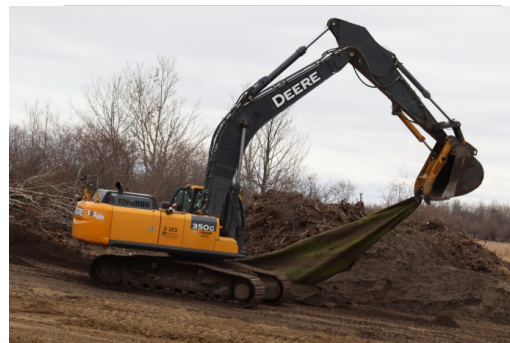
Description & Location: SSKP 817+300
