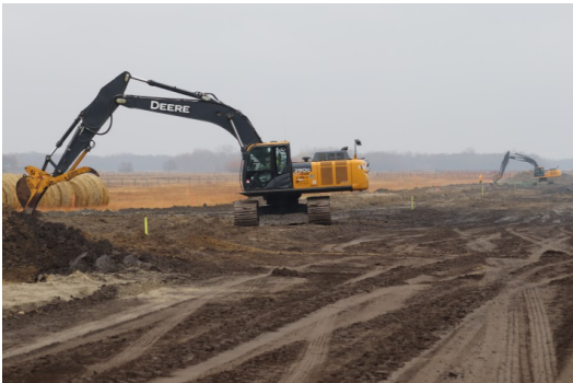
Description & Location: SSKP 831+300
