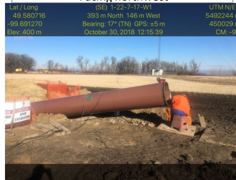
Description & Location: SSKP 907+650
