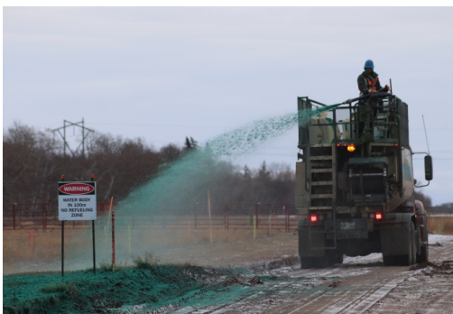
Description & Location: SSKP 857+726
