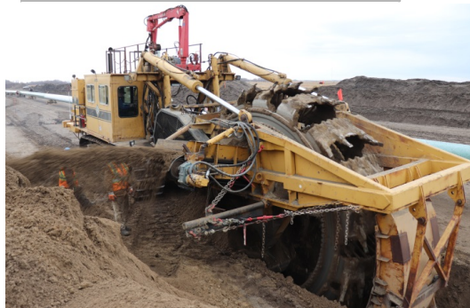
Description & Location: SSKP 837+000
