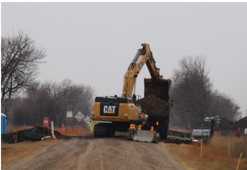
Description & Location: SSKP 860+756
