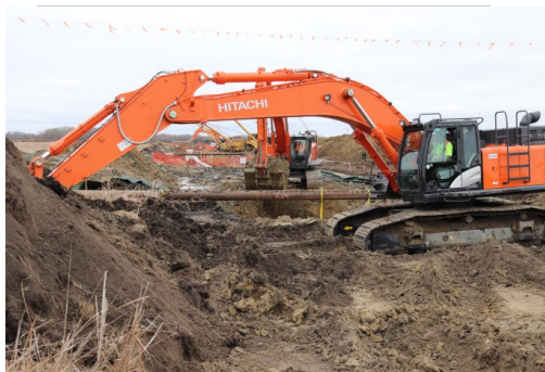
Description & Location: SSKP 821+150
