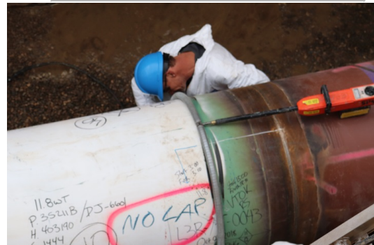
Description & Location: SSKP 827+700
