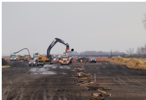
Description & Location: SSKP 810+100
