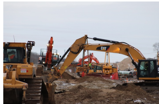
Description & Location: SSKP 842+850
