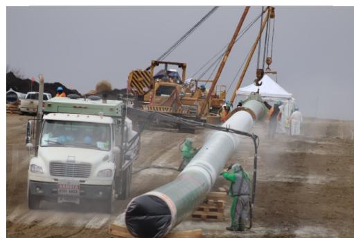
Description & Location: SSKP 877+058
