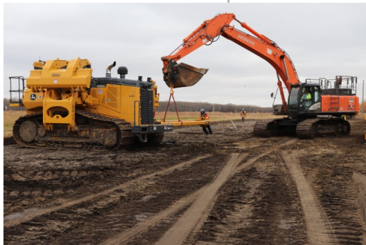
Description & Location: SSKP 841+100
